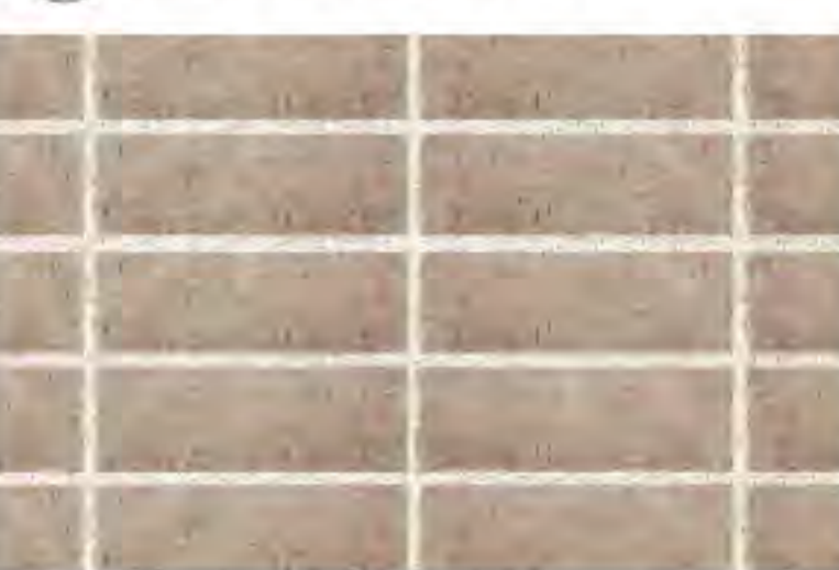
7 Podium Solid Balustrades Austral Masonry GB Honed - 'Limestone' or similar - Stack Bond
